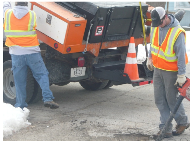
Figure 5 – Removing water & debris
