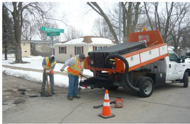
Figure 7 – Using “Patch Catch” tray for dramatically improved shoveling ergonomics
