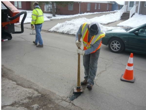
Figure 4 – Compacting material
